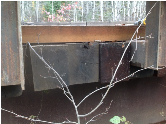
new ties added
