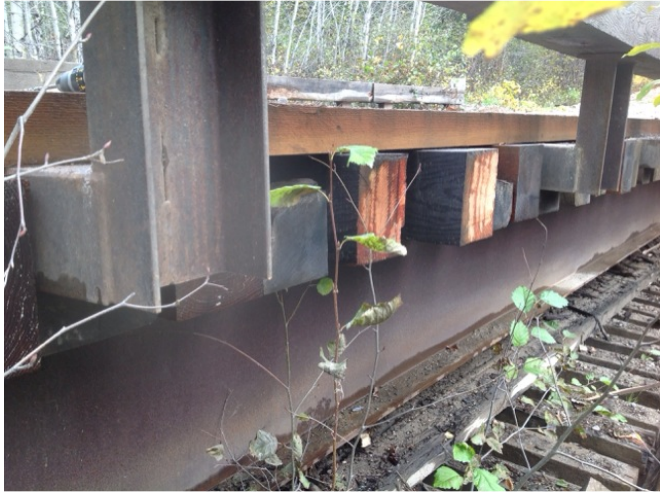
new ties added
