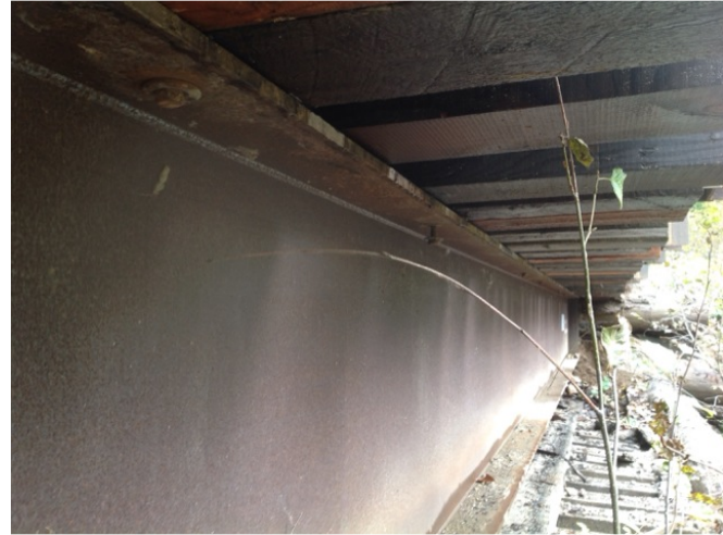
deck to girder bolts
